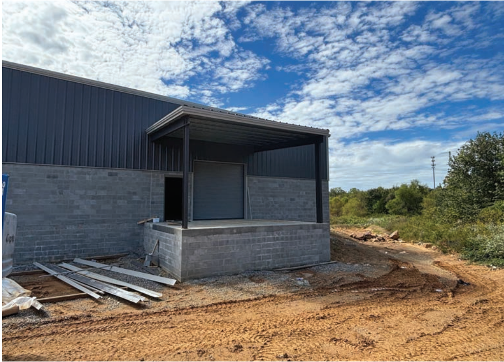
■ PHOTOS - BUILDING A
