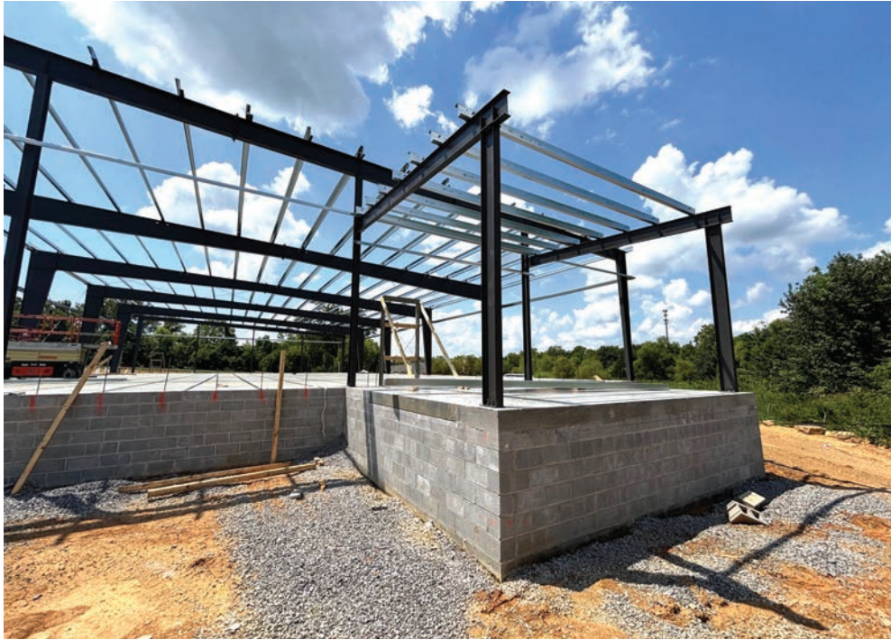
PHOTOS - BUILDING A
